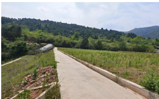
1#渣场截排水沟
